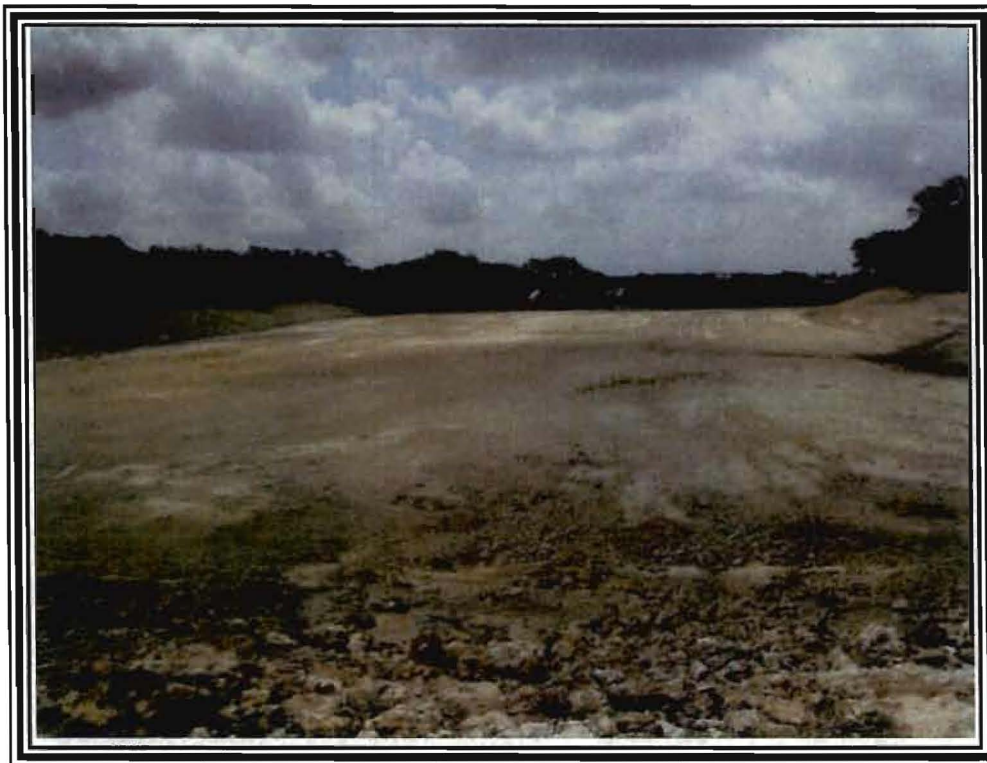
8. View of new manmade feature S-8 at Unit 09.
