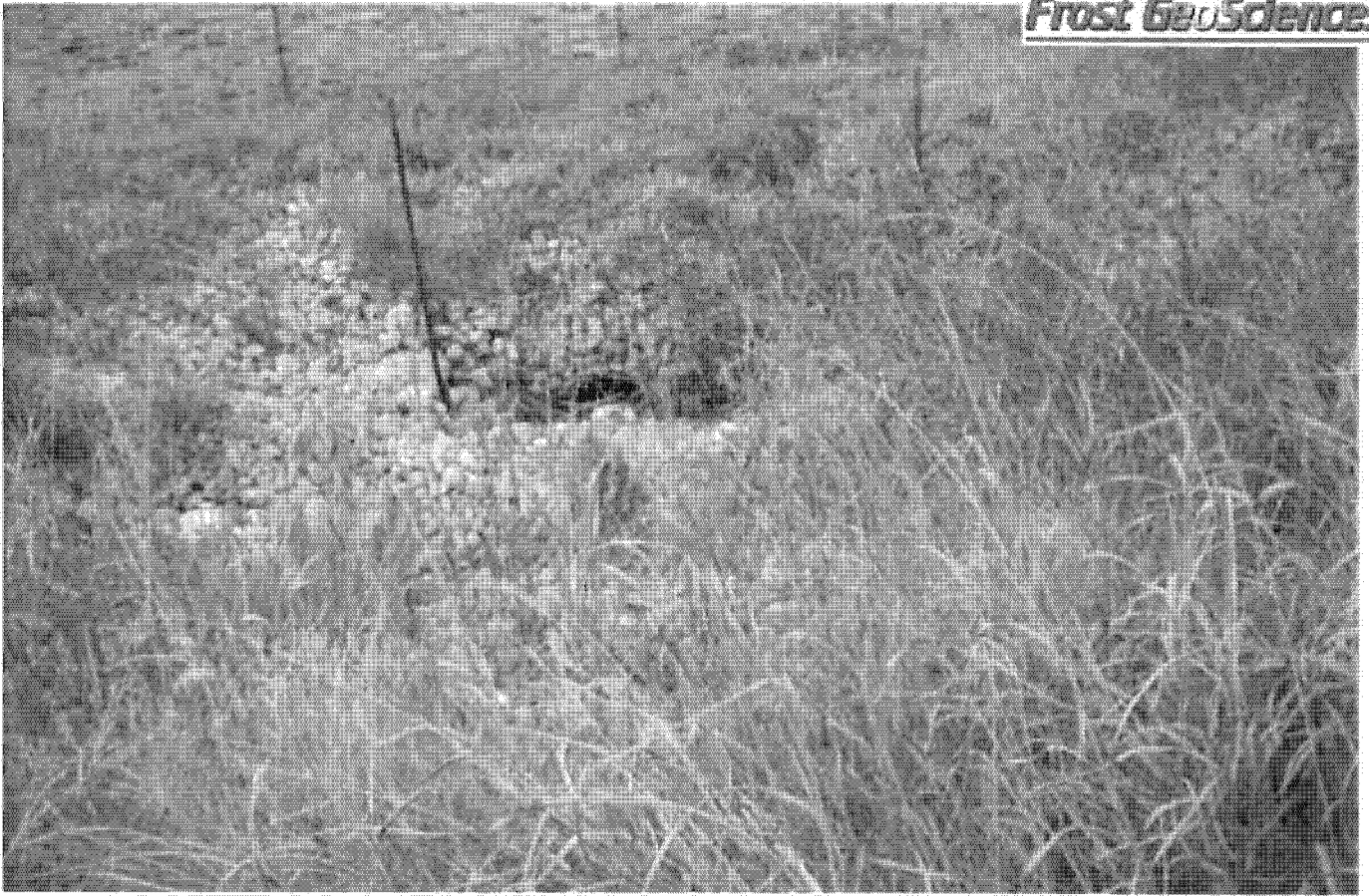
View of Potential Recharge Feature # S-1.
