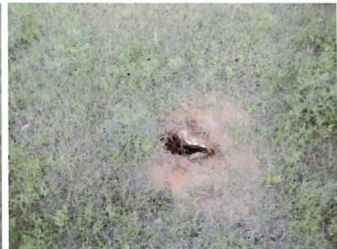
View of one of the three void openings noted as part of PRF # S-101.
