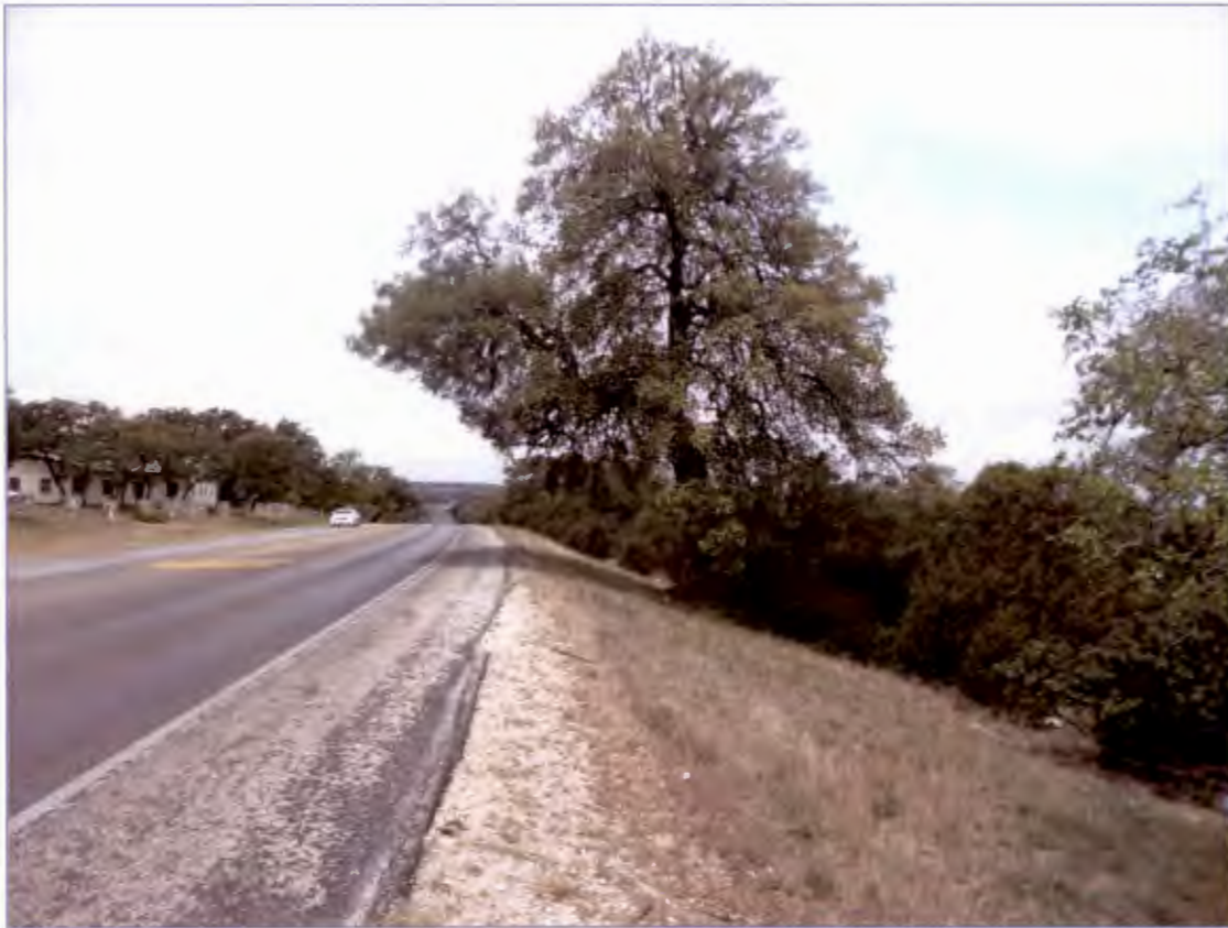
SH 46 Passing Lanes Project
