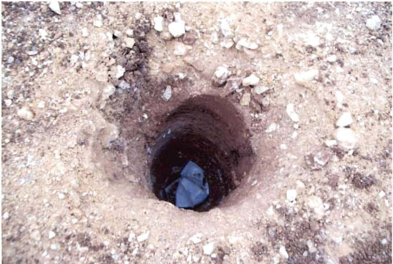
View of an excavated footing showing the depth of topsoil on a portion of Lot 47.
