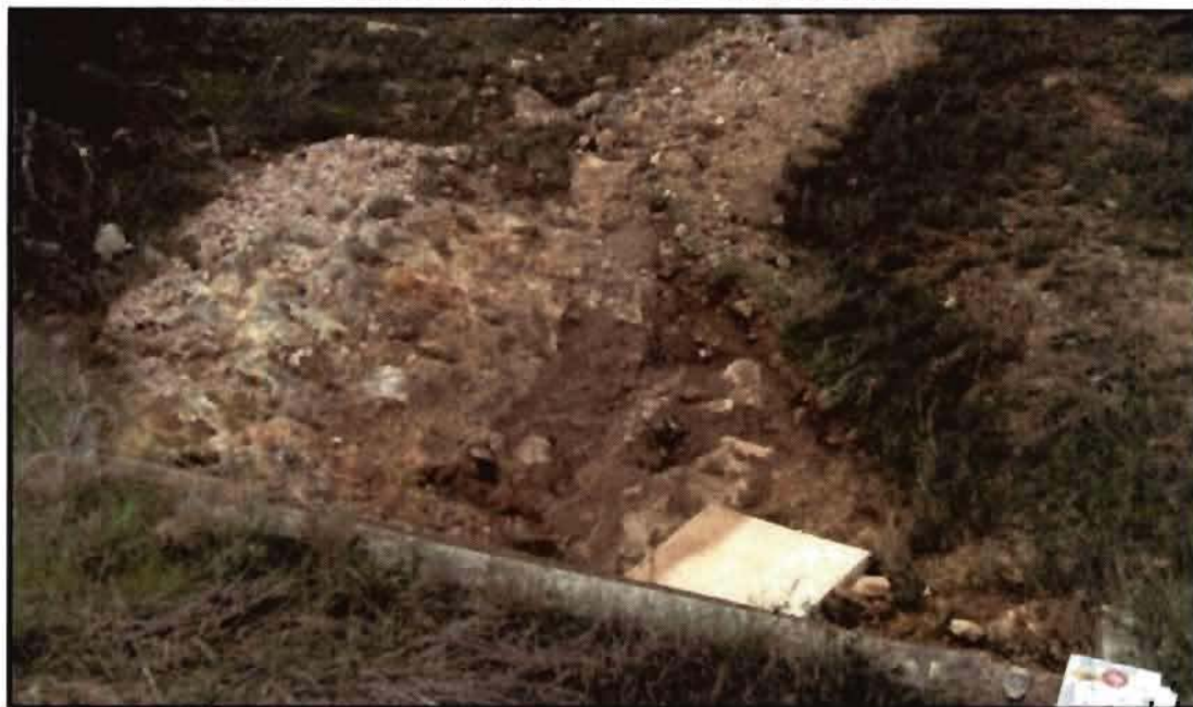
PHOTO C2 - Feature F-1. Scoured "swallow hole" at discharge end of stormwater culvert beneath FM-306. Edwards (Kainer Formation?) exposed in "hole". View towards downstream (southerwesterly). Note "terra-rosa" soil in scoured hole.
