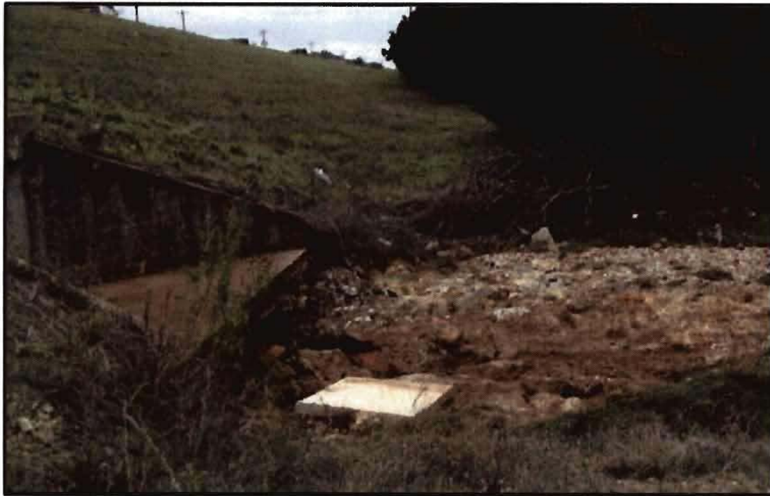
PHOTO C1 - Feature F-1. Scoured "swallow hole" at discharge end of stormwater culvert beneath FM-306. Flow to right (southwesterly). Edwards (Kainer Formation?) exposed in "hole". View to south.
