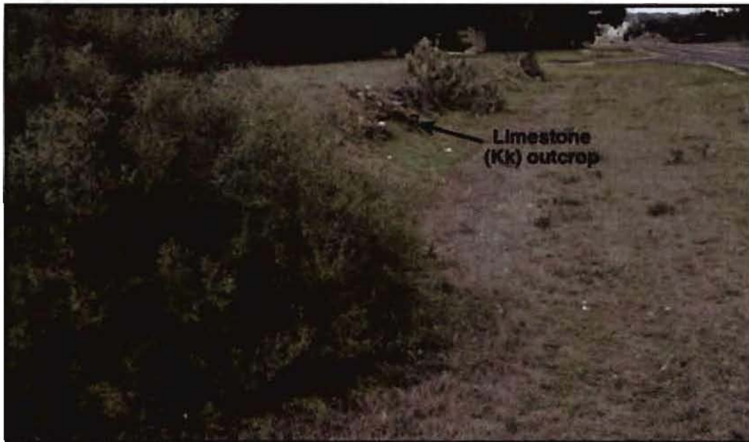
PHOTO E1 - View to north from near southern end of Site. FM-306 at right, Privacy and residential subdivision to left. View is along ROW, graded to direct runoff away from homes. Cut/grading exposed limestone (Kk) outcrop in upper foreground
