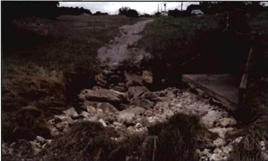
PHOTO D1 - Feature F-2. Scoured "swallow hole" at discharge end of stormwater culvert beneath FM-306. Flow to left (southwesterly). Edwards (Kainer Formation?) exposed in "hole". View to north. Note concrete "paved" ROW channel draining towards F-2.
