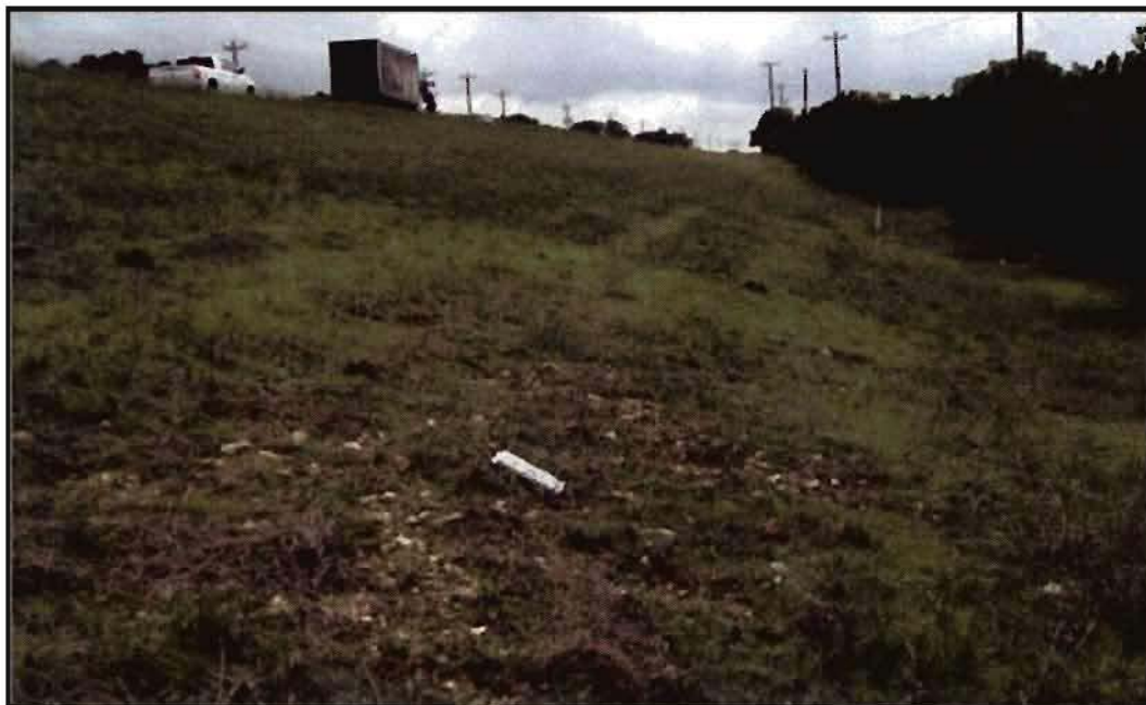
PHOTO F1 - Typical cut/filled/graded ROW along southern half of site. FM-306 to the left. Gravel/cobbles visible in foreground appear to be imported, as part of ROW channel construction. Scarce bedrock outcrops and in-situ soils. Channel thalweg near tree-line at right.
