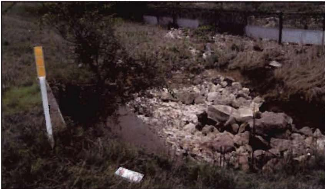
PHOTO D2 - Feature F-2. Scoured "swallow hole" at discharge end of stormwater culvert beneath FM-306. Edwards (Kainer Formation?) exposed in "hole". View towards downstream (southerly). Culvert & FM-306 to the left.
