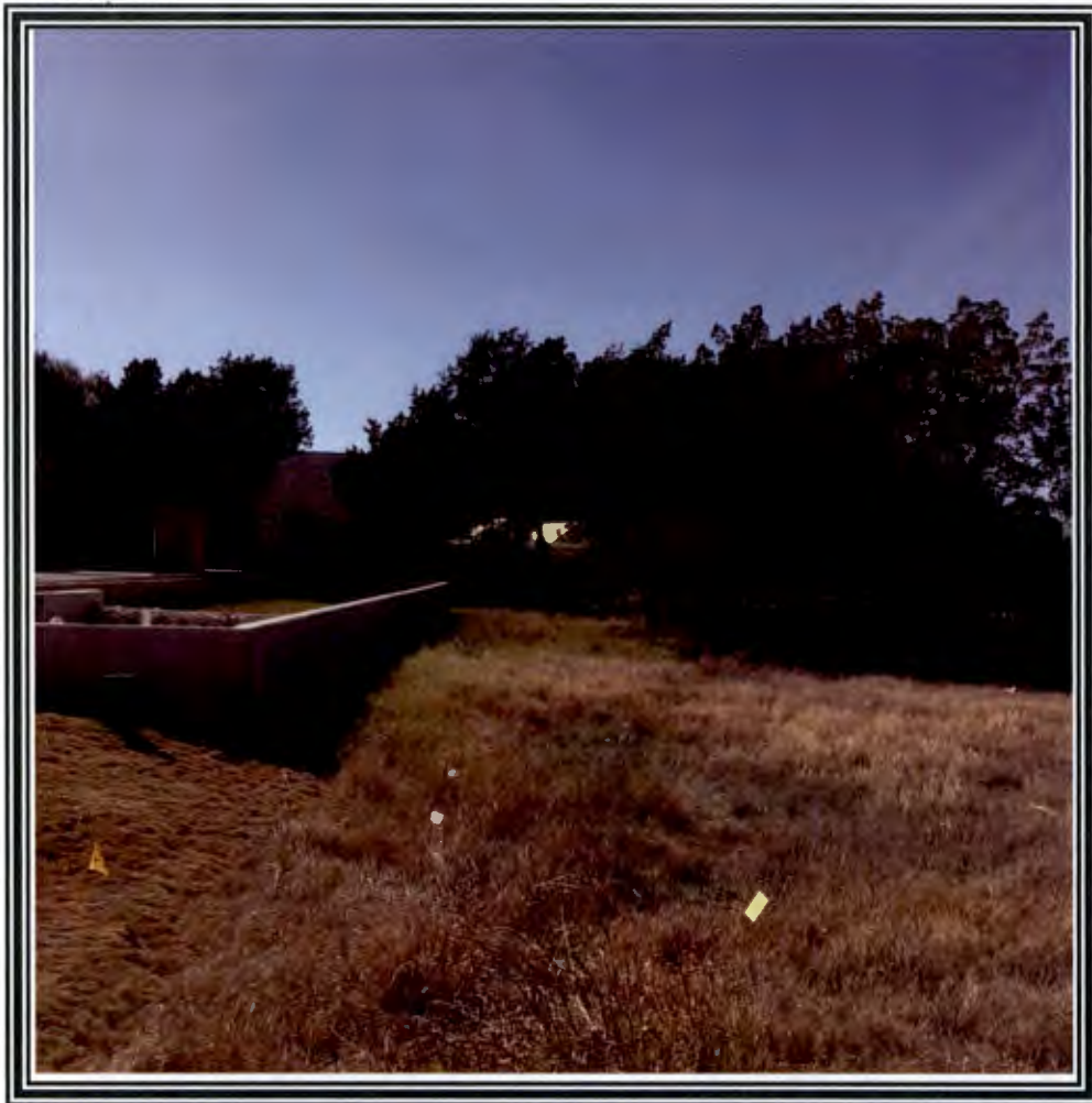
8. View south along the east property line from the northeast corner. Note storm water retention structure on the east adjacent property.
