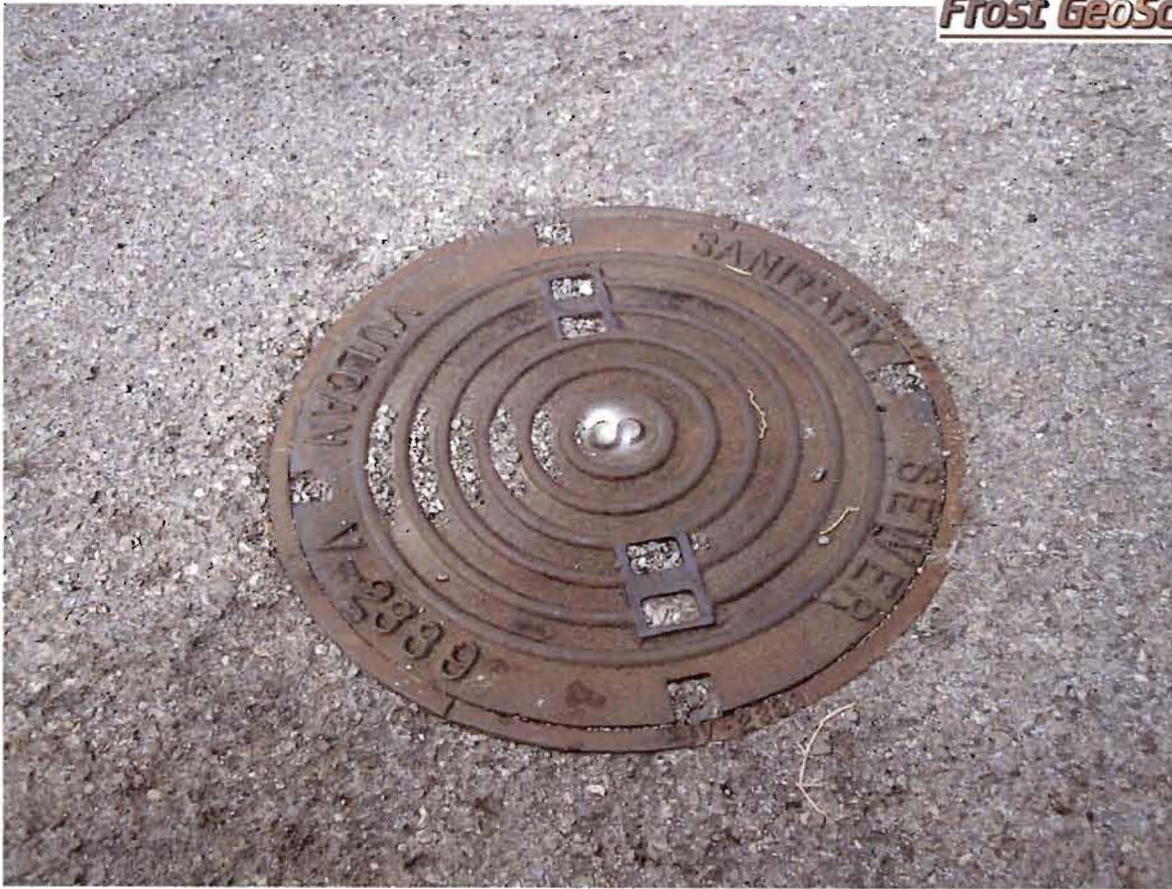
View of Potential Recharge Feature (PRF) #S-3.
