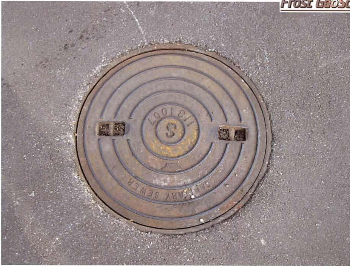
View of Potential Recharge Feature (PRF) #S-1.
