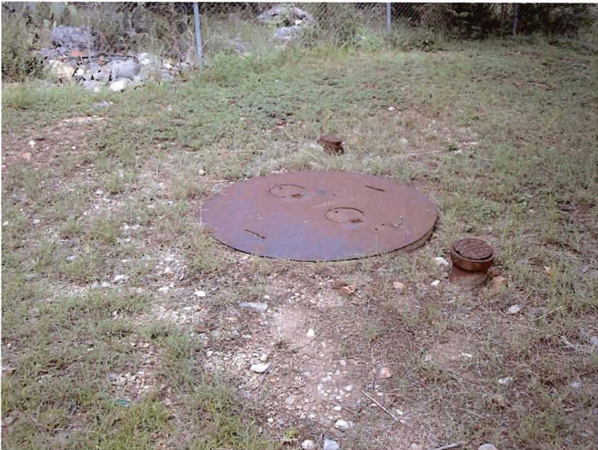
View of Potential Recharge Feature (PRF) #S-6.
