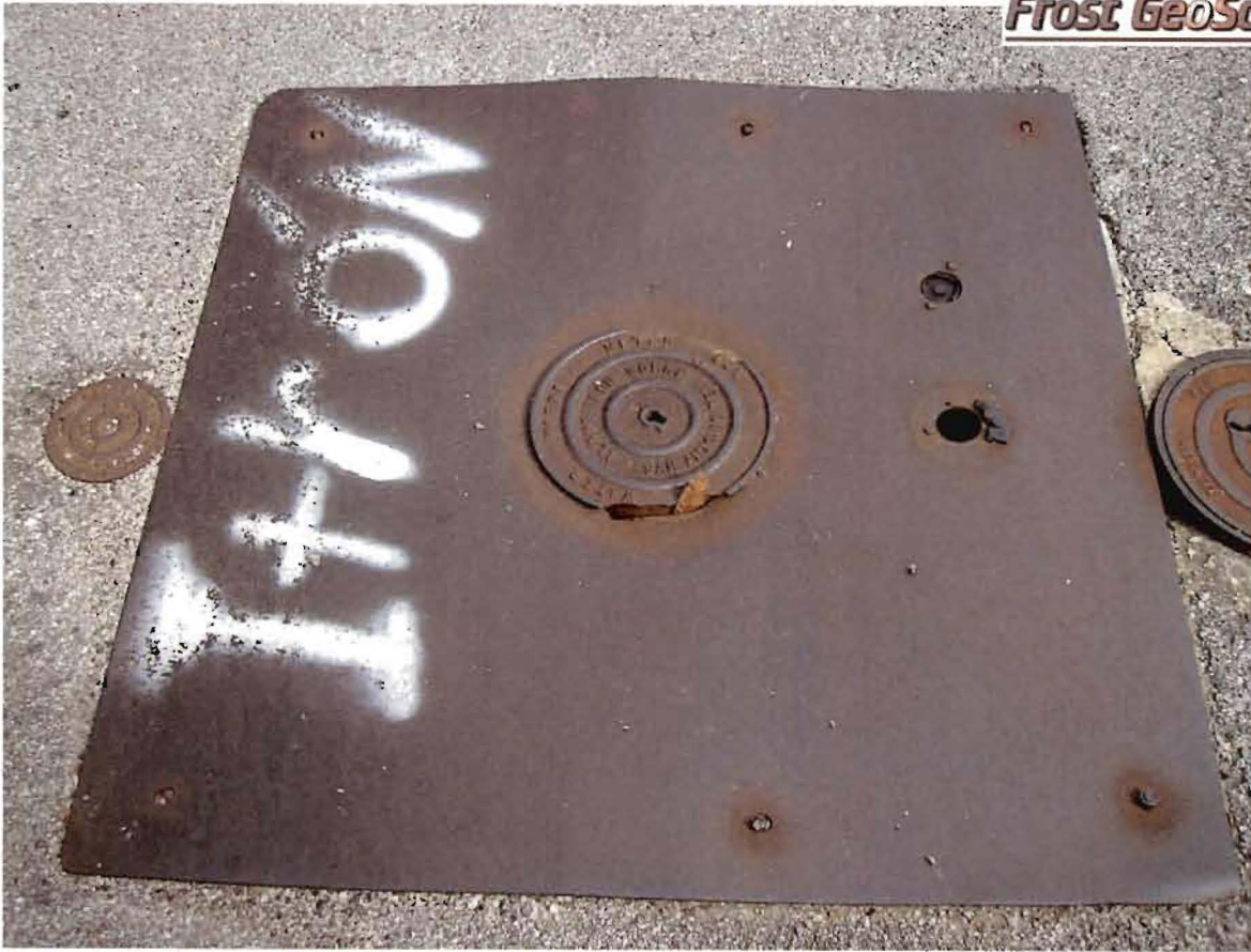
View of Potential Recharge Feature (PRF) #S-7.
