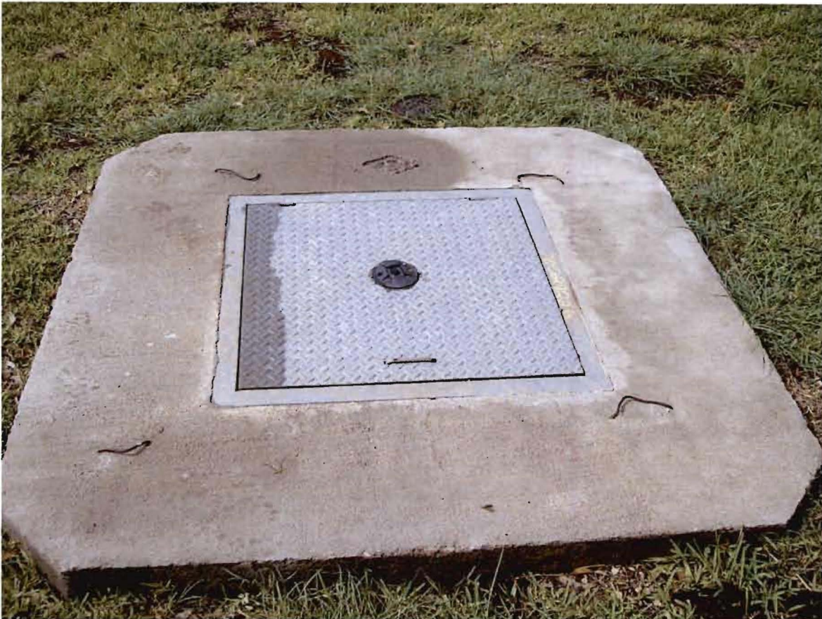
View of Potential Recharge Feature (PRF) #S-8.
