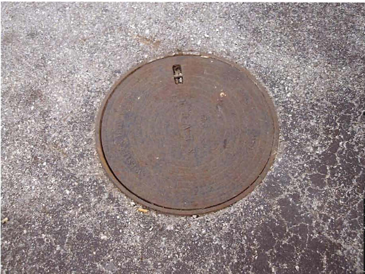
View of Potential Recharge Feature (PRF) #S-4.
