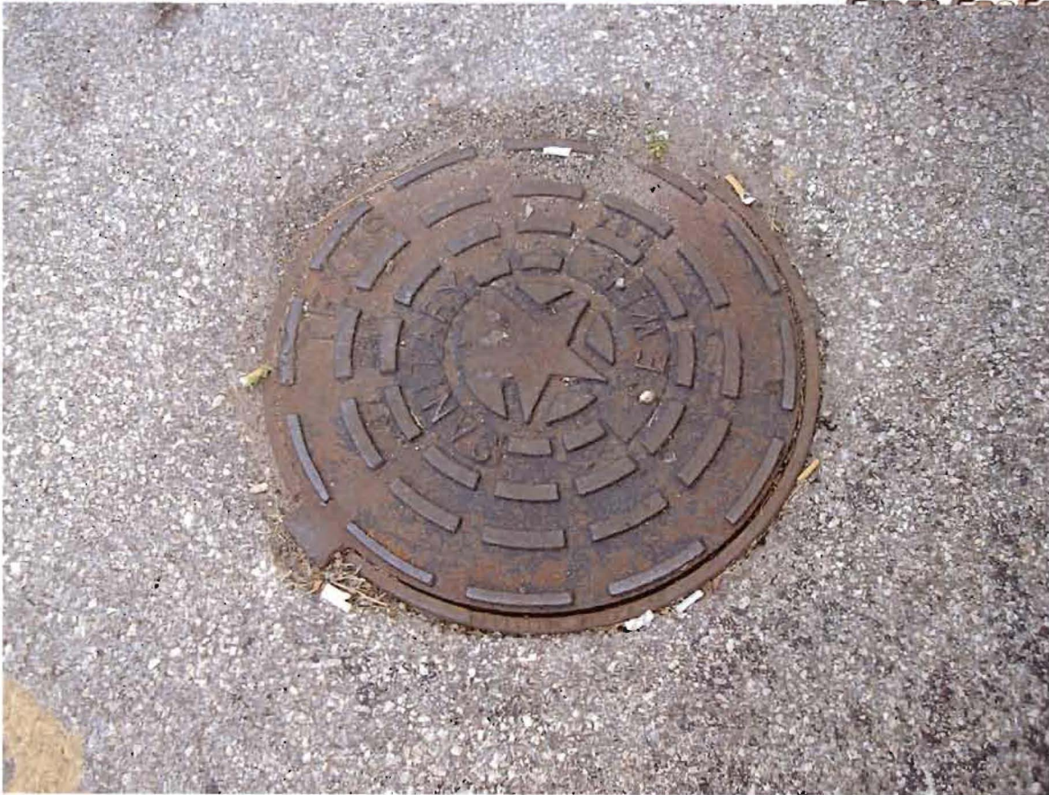
View of Potential Recharge Feature (PRF) #S-5.
